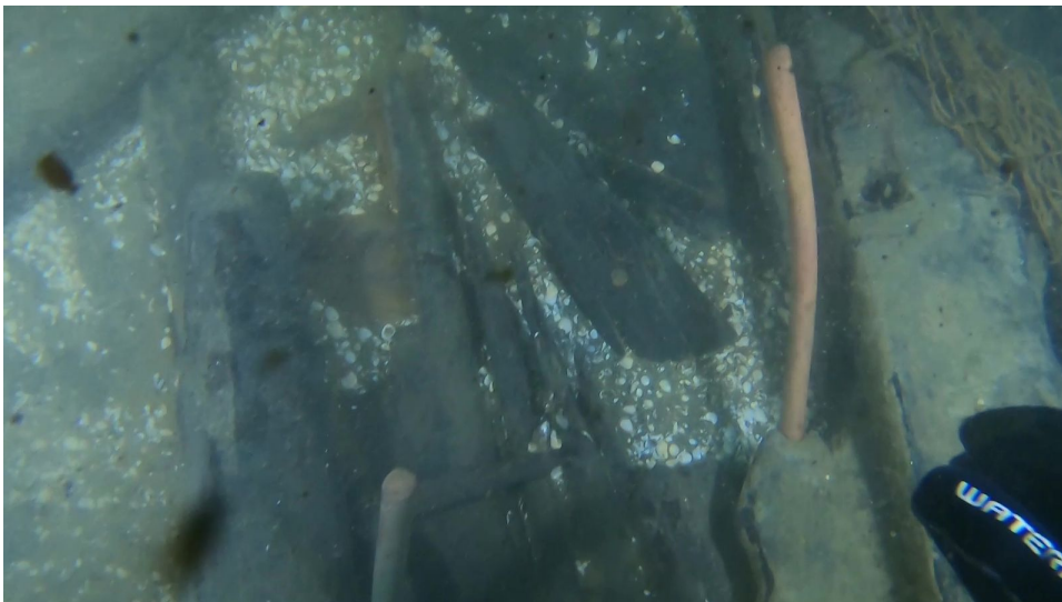
Massive copper rods / connectors
